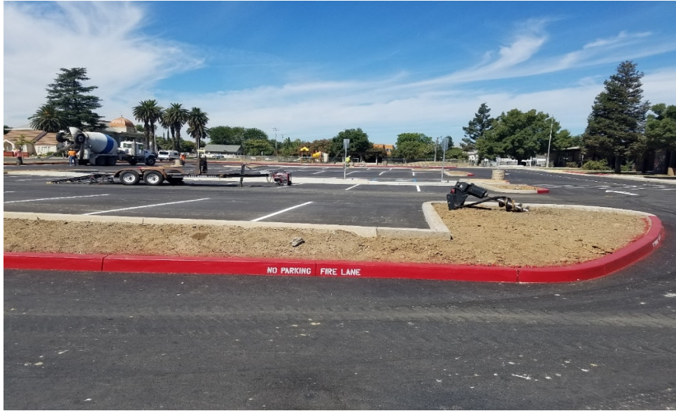
New Parking Lot in front of School
